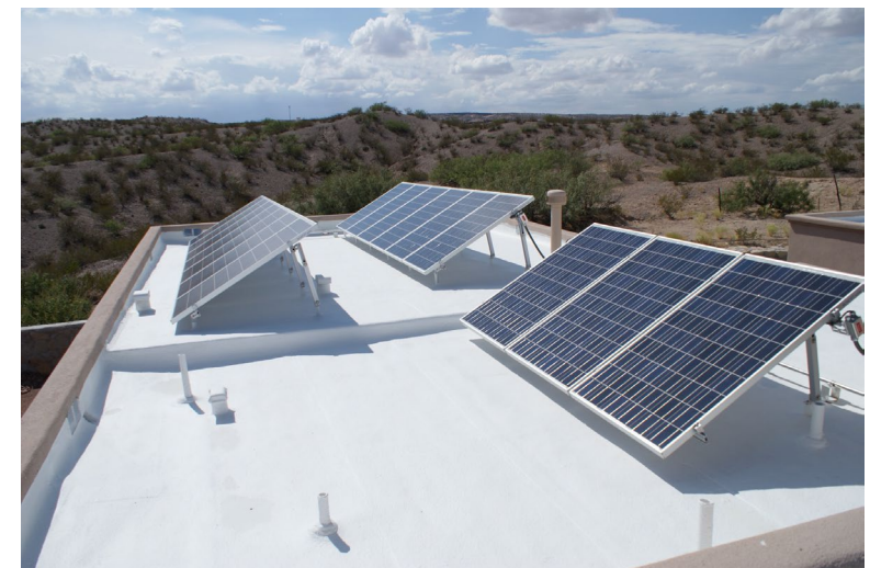
Credit: Carlisle Roof Foam
