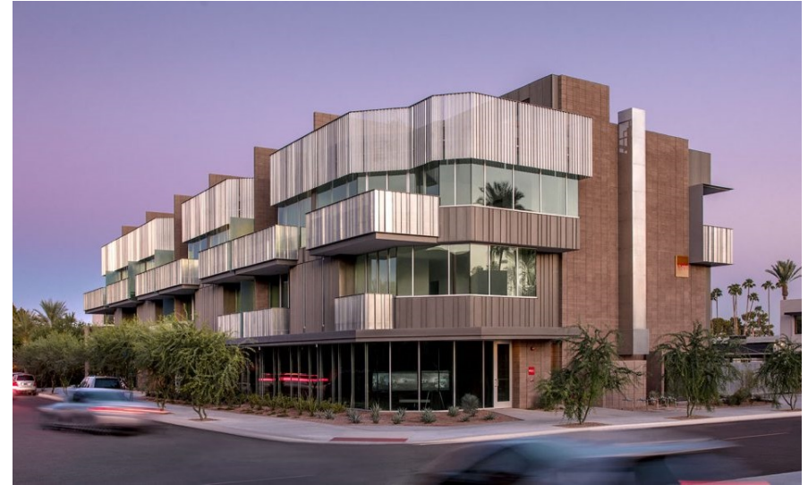
Eldorado on 1 st Condos – Will Bruder Architects
