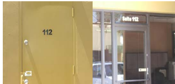
Suite numbers should be clearly marked on both front and rear doors.
