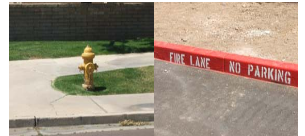
Unobstructed Fire Hydrant
