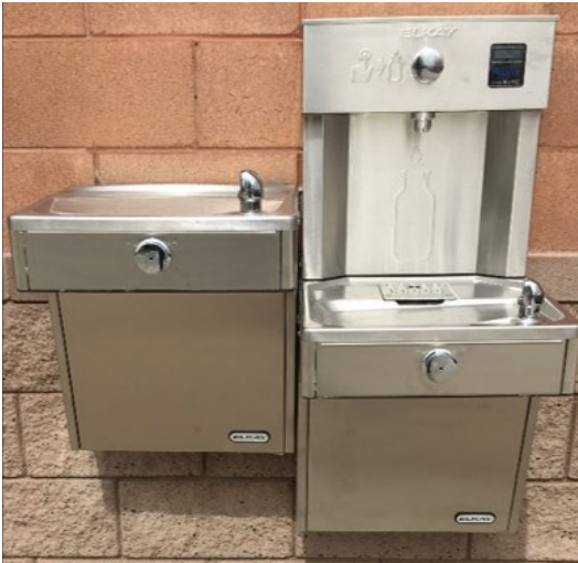
Newly installed drinking fountain replacement
