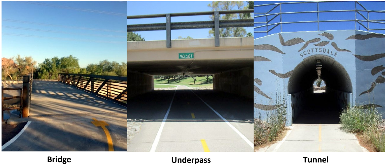
Figure P-6: Grade Separated Crossings
